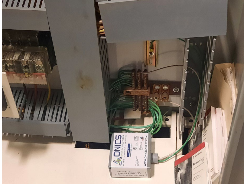
Figure 8: Onics installation on ground in drive panel.
